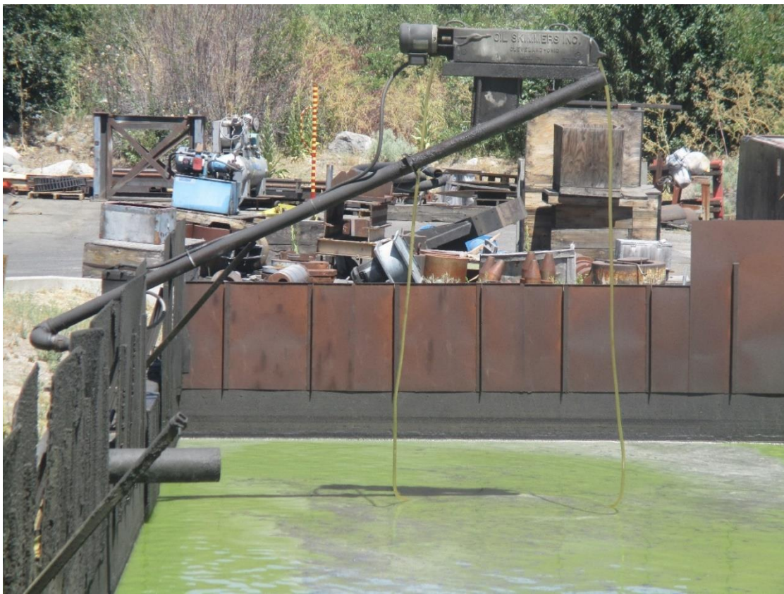
Figure 14 - Oil skimmer in Shop Pond
