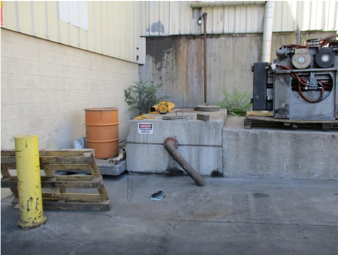
Figure 8 - Recycled water systems clean out box
